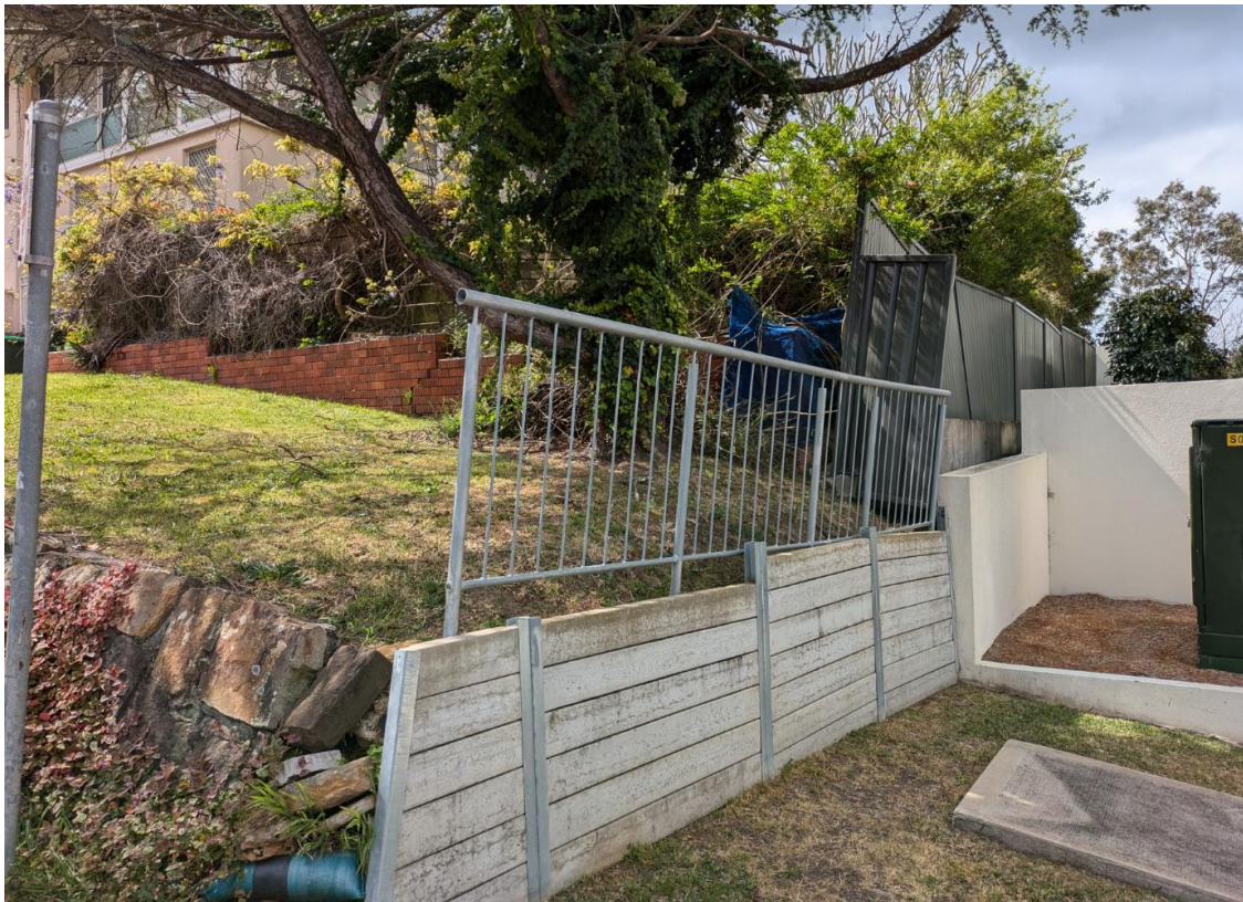
Image 2: Retaining structure across the southern portion of site
