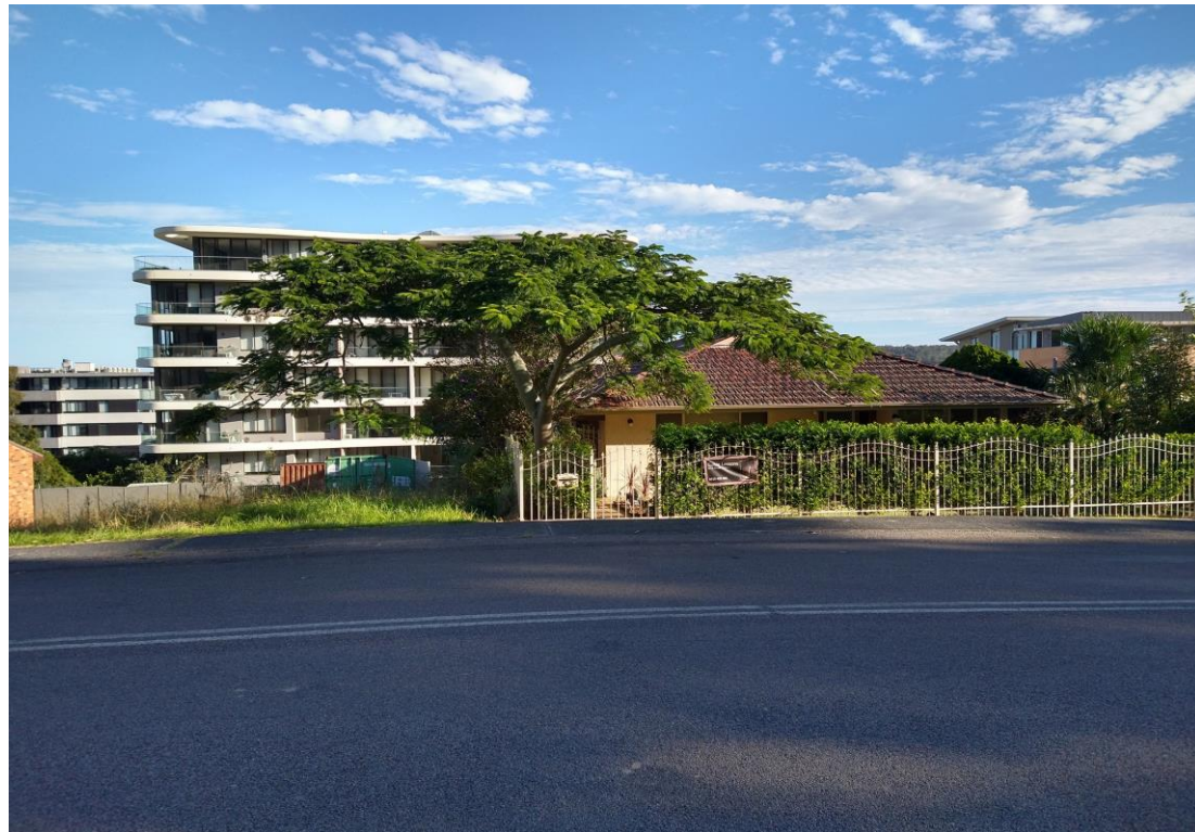
Photo 2 - Site, looking toward the south, 15 April 2021.
